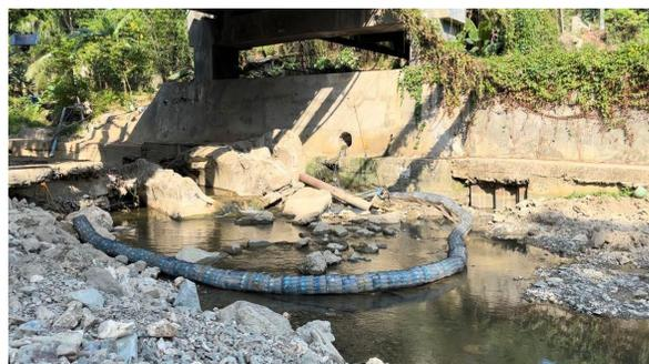
**Figure 4.** Biofence located in the Butuanon River Upstream in Barangay Pit-os.
